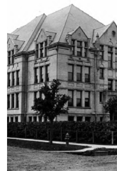
Fig 9. North Community High School, Minneapolis, Minnesota, 1914–73. Beal attended the school in the 1890s.
